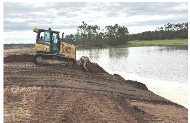
Active dirt backfilling of construction pond.
